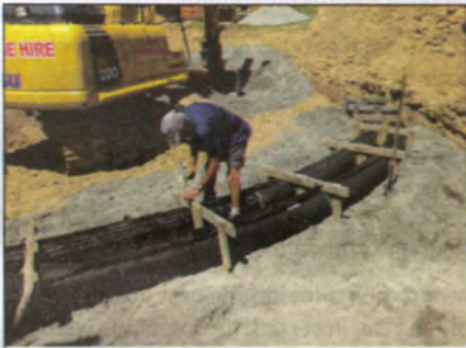
Onuku Marae installation
